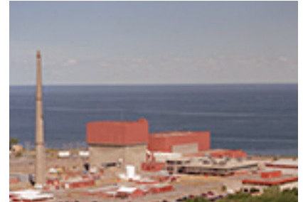
FitzPatrick Nuclear Power Plant
